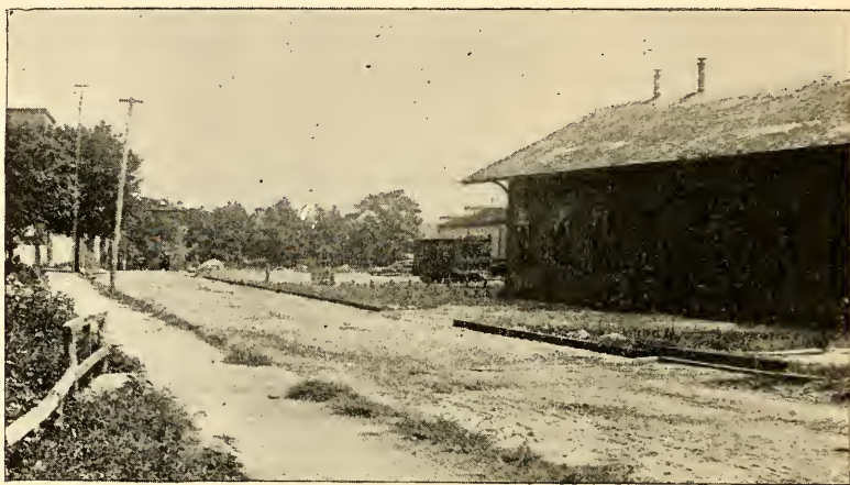
57. The Fatal Bridge, in foreground looking towards Princess Anne St.—Old R. R. Depot seen beyond the car at right, 1891.
